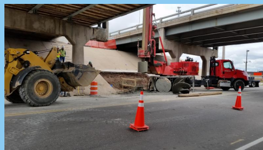
Indiana Bridge under construction
